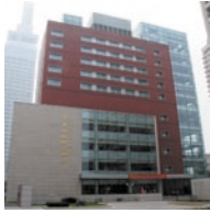
New Building of the Center
