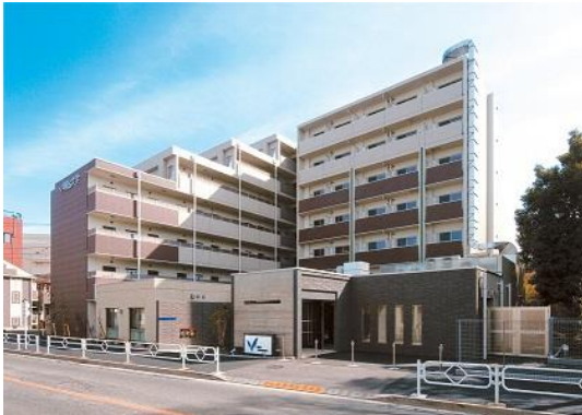
Exterior of the building
